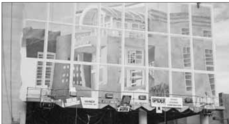
© Mark Switlik, work in progress circa 1992, Mural for the Phoenix Suns
